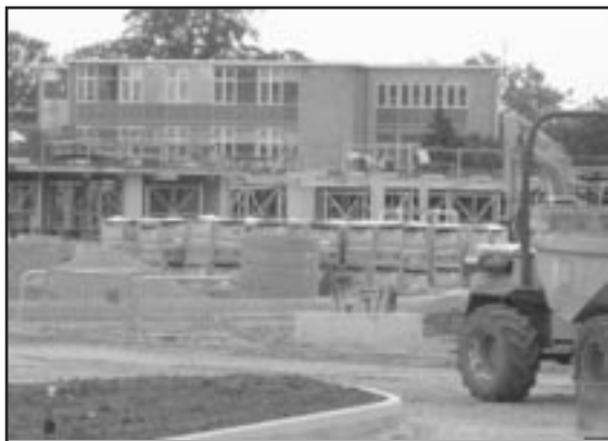
Kingsmead School with construction for new Academy
