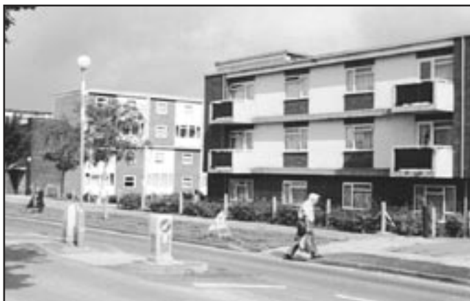
Sochi Court flats which were demolished in 2003 (DE 2001)
